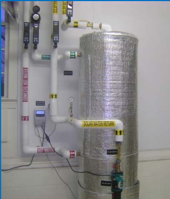
Solar Thermal Drain Back Tank & Piping
